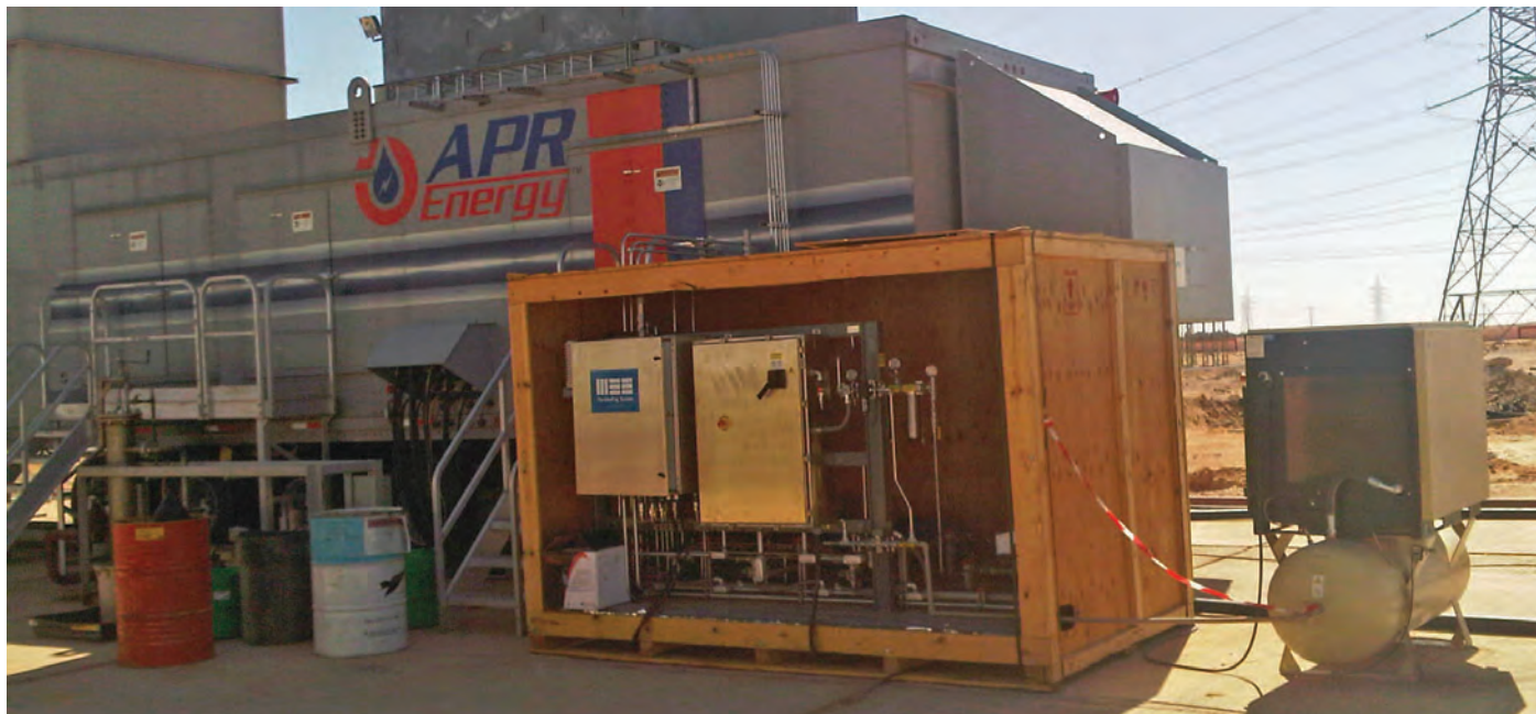
Fog skid deployed at APR Energy site on Pratt and Whitney FT8 MobilePac gas turbine in Libya. Courtesy of Mee Industries
