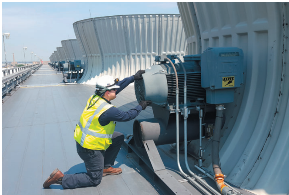
Any reconstruction effort should begin with an inspection of the cooling tower by an experienced cooling tower service provider. The scope of work should be defined by their findings and recommendations.
