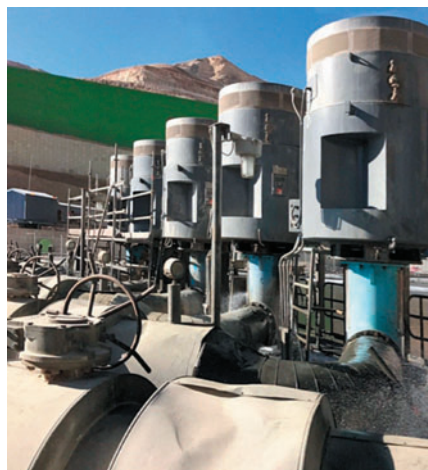
New two-stage pumps for solids handling
