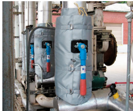
Insulation blankets inhibit corrosion by preventing water ingress
