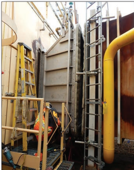
Figure 5: New hot-to-cold transition duct
