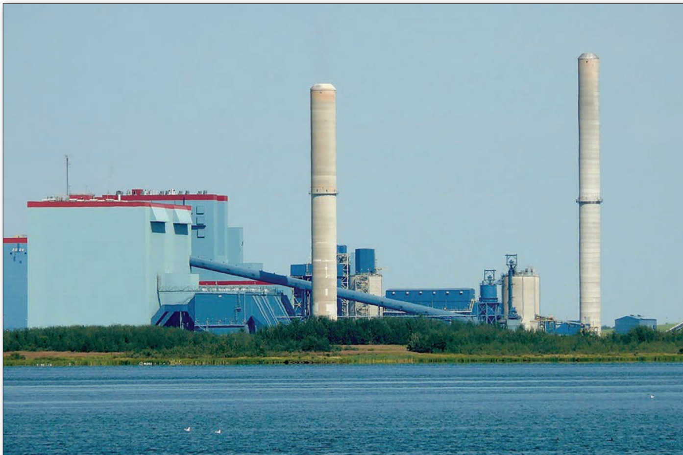
Figure 2: Expansion of the Genesee Power Plant in Alberta, Canada is currently taking place using the MHPS M501J gas turbine in a single-shaft combined cycle configuration. This is said to result in a reduction in building size and cost savings
