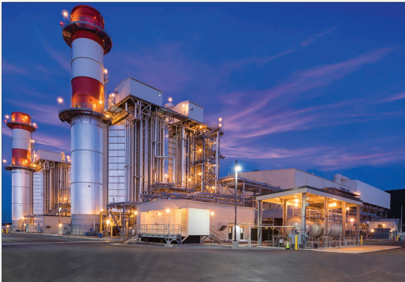
Figure 5: Siemens H-class technology has been deployed at the Patriot and other plants in the U.S. in a single-shaft configuration
