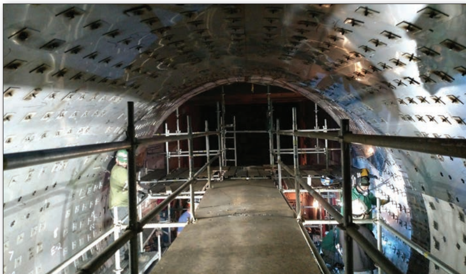
Figure 3: New liner system with carefully spaced studs
