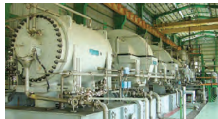
Steam turbine in ethylene service (Courtesy of Elliott Group)
