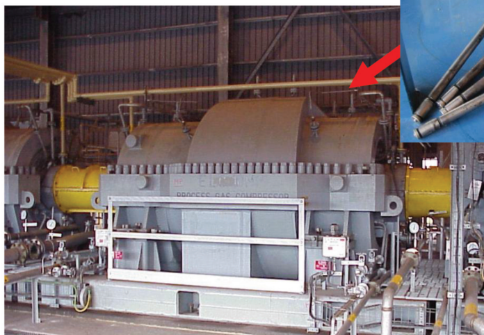
Figure 5. Water injection nozzles are located on the casing in order to be able to inject the water spray into the compressor stages.
